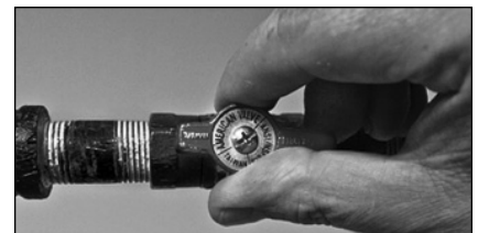
Figure 58 - Gas valve in “on” position.
