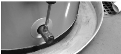
Figure 42 - Draining the water heater.
