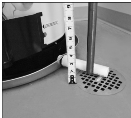
Figure 26 - Temperature and Pressure Relief Valve Pipe
