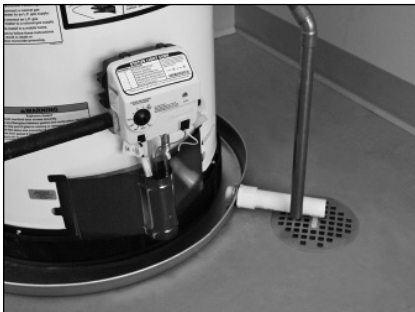
Figure 23 - Metal drain pan piped to drain.
