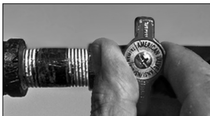
Figure 50 - Gas valve in “off” position.
