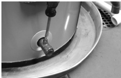
Figure 20 - Draining the old water heater.
