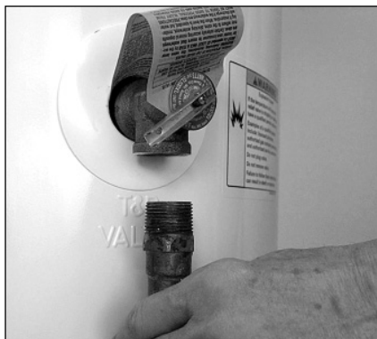
Figure 21 - Removing the T&P Relief Valve discharge pipe.
