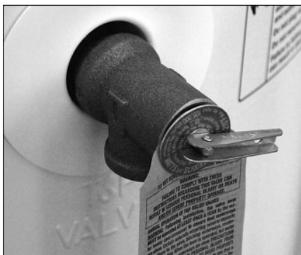
Figure 25 - Temperature and Pressure Relief Valve
