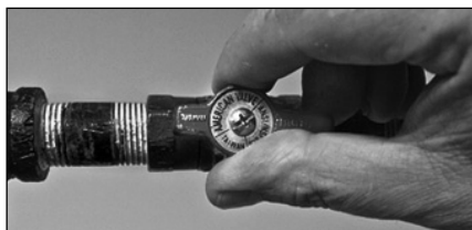
Figure 32 - Gas valve in "on" position
